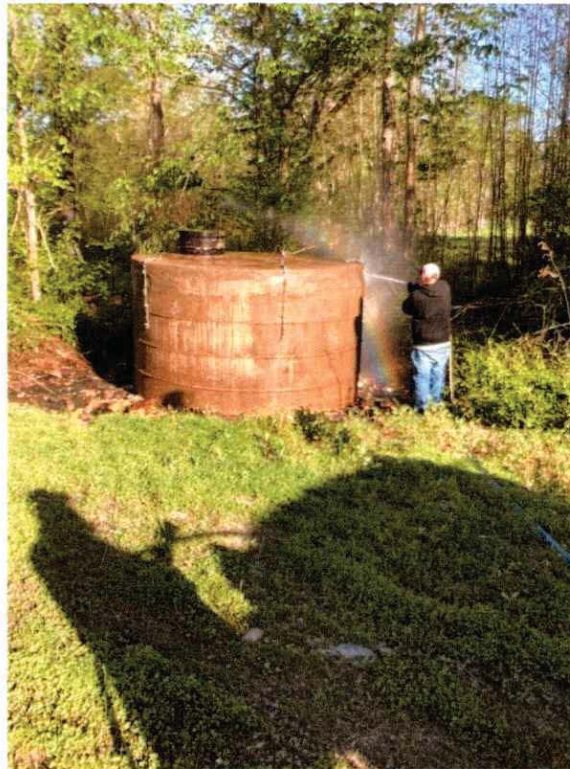
MH 1865 During cleanup 4/6/2025
