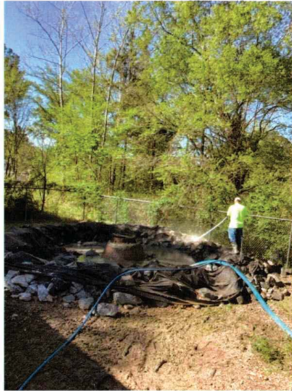
MH 1865 During cleanup 4/6/2025
