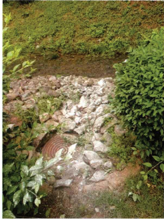
MH 3728 After cleanup 4/6/2025
