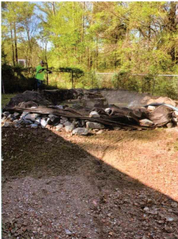
MH 1866 During cleanup 4/6/2025
