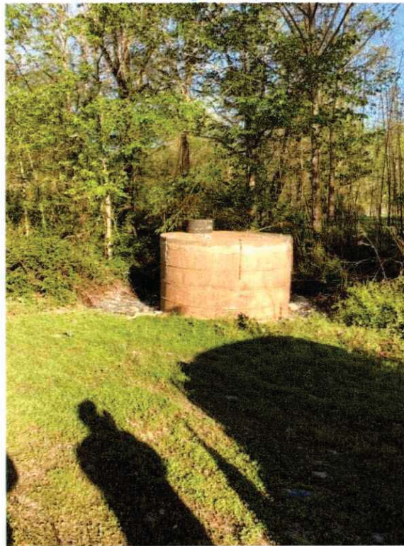
MH 1865 After cleanup 4/6/2025
